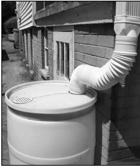
Rain barrels serve dual purposes: they help prevent excessive stormwater runoff that can damage streams and provide free irrigation water for home landscapes.
