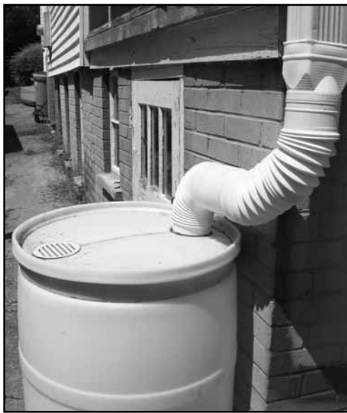
Rain barrels serve dual purposes: they help prevent excessive stormwater runoff that can damage streams and provide free irrigation water for home landscapes.
