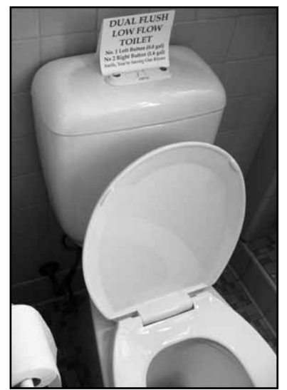
High efficiency toilets like this one will be required in new construction after July 2012 under Gov. Sonny Perdue's water conservation bill. This one's in Executive Director Joe Cook's house...call for demonstrations!
