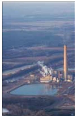
The report also calls on Georgia's Environmental Protection Division to require Georgia Power Co. to install a modern cooling-water system at Plant Hammond. Built before passage of the Clean Water Act in 1972, the plant still uses the "once-through" cooling system constructed when the facility opened in 1954. Modern power plants use closed systems that require considerably less water.
