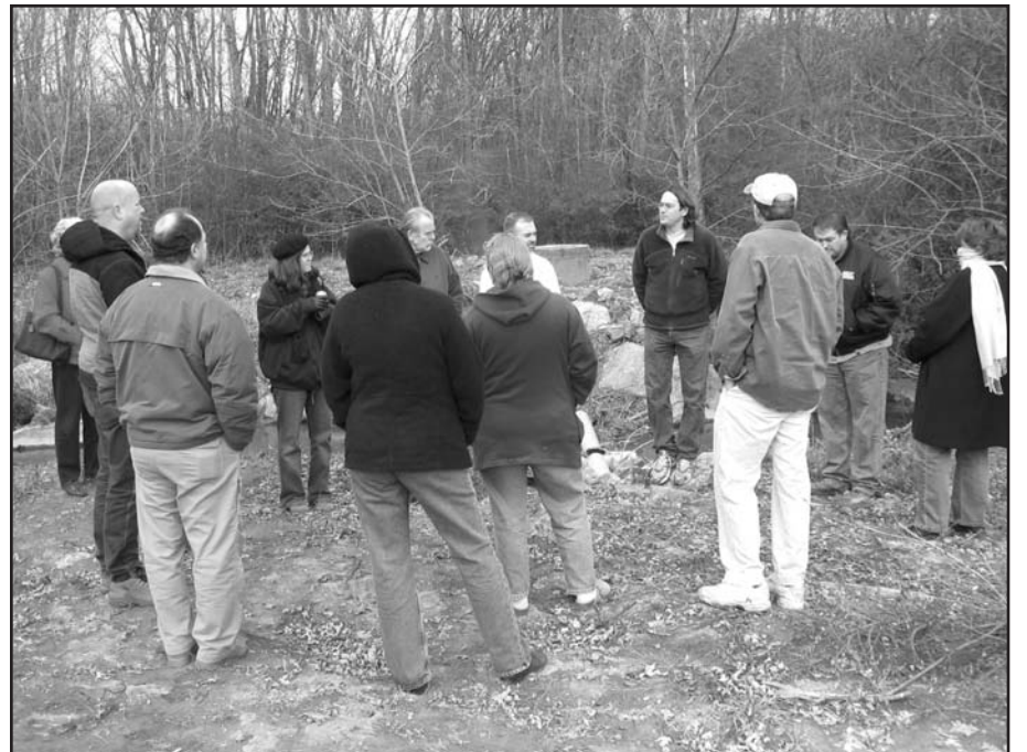
Get the Dirt Out workshop participants tour a construction site in Calhoun.
